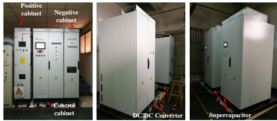
Fig. 23. Photos of the MW level energy storage device.
